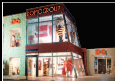
Domogroup exclusive showroom
